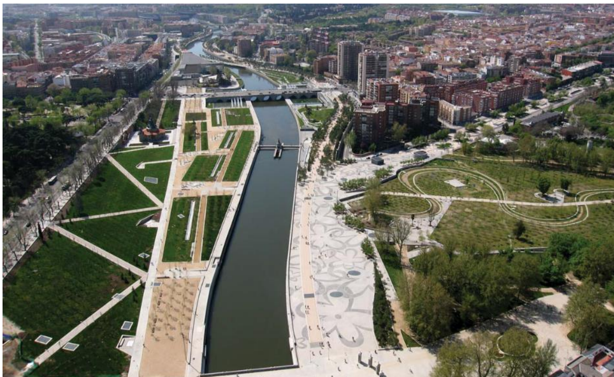
Figura 139 – River Regeneration Project, Madrid Río, Spain
